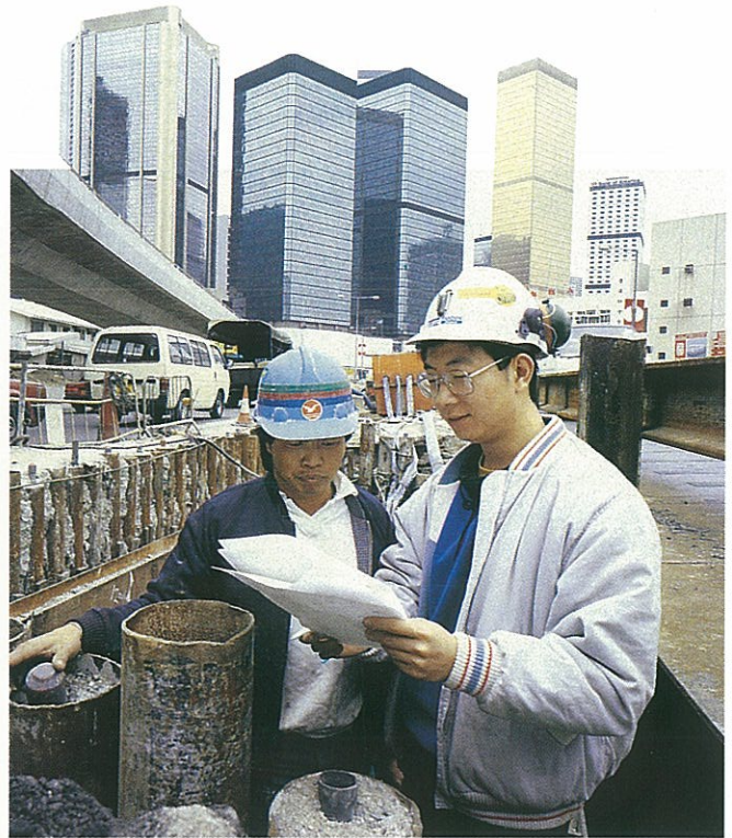
Hongkong. Kent Chan (right) visits a contractor who is using our TUBEX method for a job of civil engineering.
