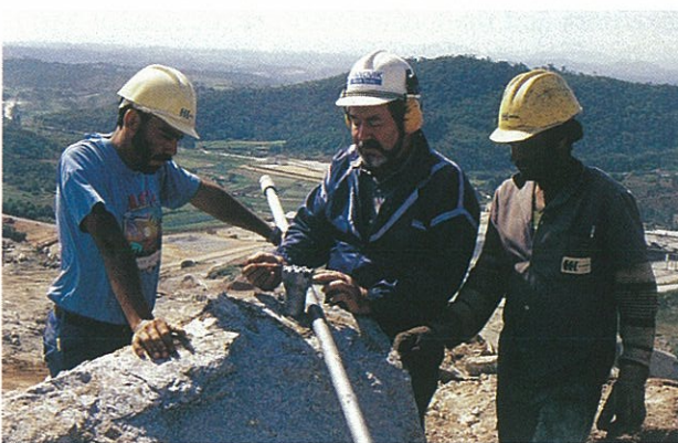
Brazil. Ataliba Ramalho Filho on site with Sandvik equipment for production drilling.
